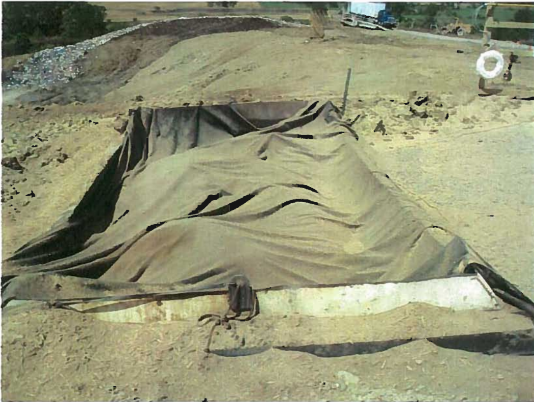
Date: 4/18/2012 Time: 11:08 A.M. Direction: west Photo by: S. Williams Exposure #: 007 Comments: unsecured tarp on solidification container & sawdust on the ground
