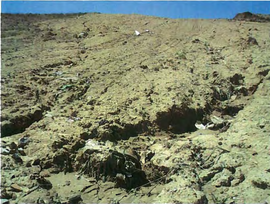
Date: 4/18/2012 Time: 12:02 P.M. Direction: southwest Photo by: S. Williams Exposure #: 011 Comments: exposed refuse amid erosion gullies
